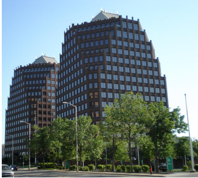
AMERICAN CENTURY TOWERS
